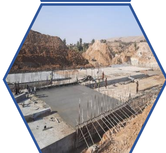
Sindh Resilience Project, Small Dam Sehwan
