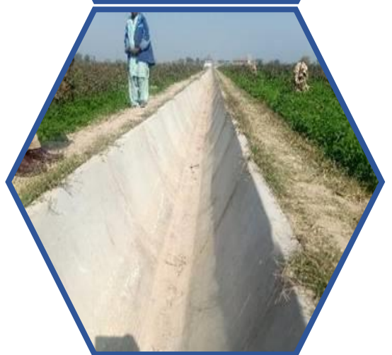
Lining of Water Course Matliari
