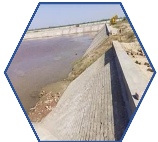
Pipe Line Water Supply Kunri Distt. Tharparkar
