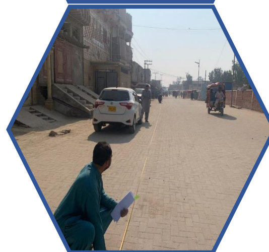
Paver work in various roads at Jacobabad
