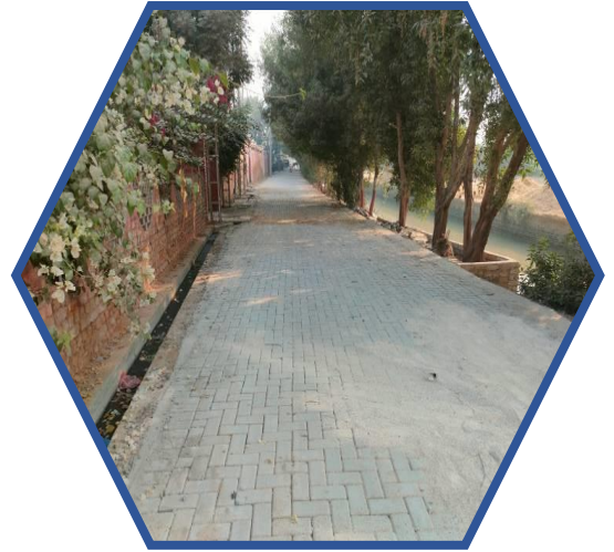
Paver Blocks for Muhallas of Shahdadkot City
