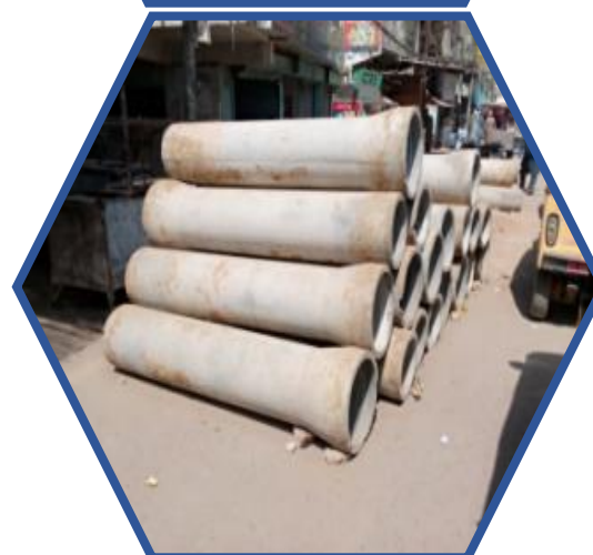
Sewerage Line, Paver Block and Carpeting Road UC-3 Karachi
