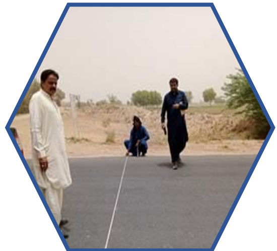
Link road from National Highway Thatta City
