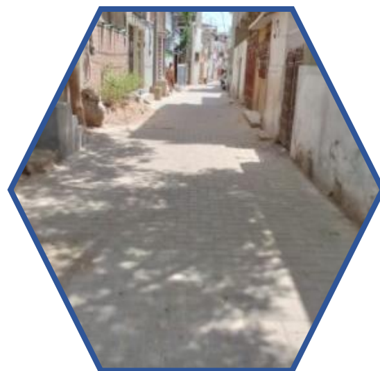
Paver Block Work in UC-17, 27 & 28 at Karachi
