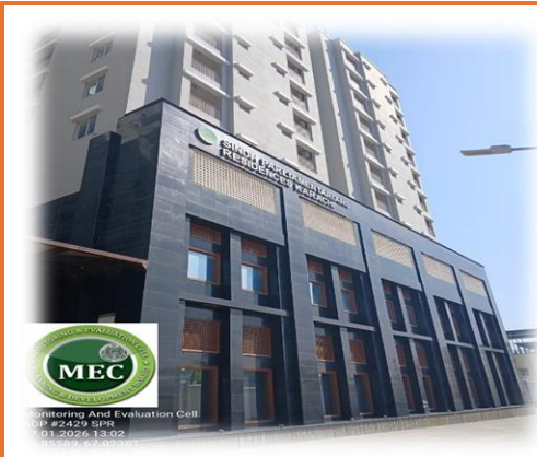
Construction Of Sindh Parliamentarian Residences
