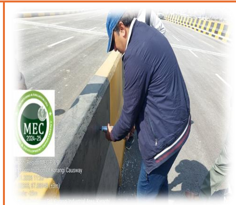
Korangi Causeway Bridge NDT through Schmidt Hammer
