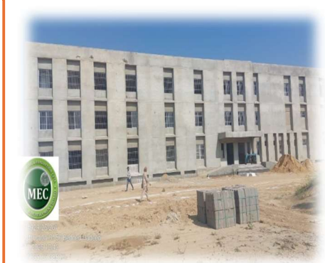
Visit of Construction of 50 Bedded Hospital at Gulshan-e-Hadeed Karachi
